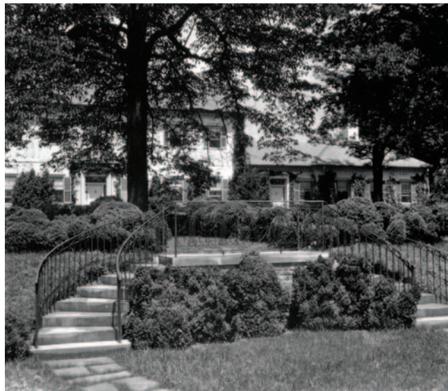
Fig. 2: Front of Chatham looking east with Music Stair in foreground.
