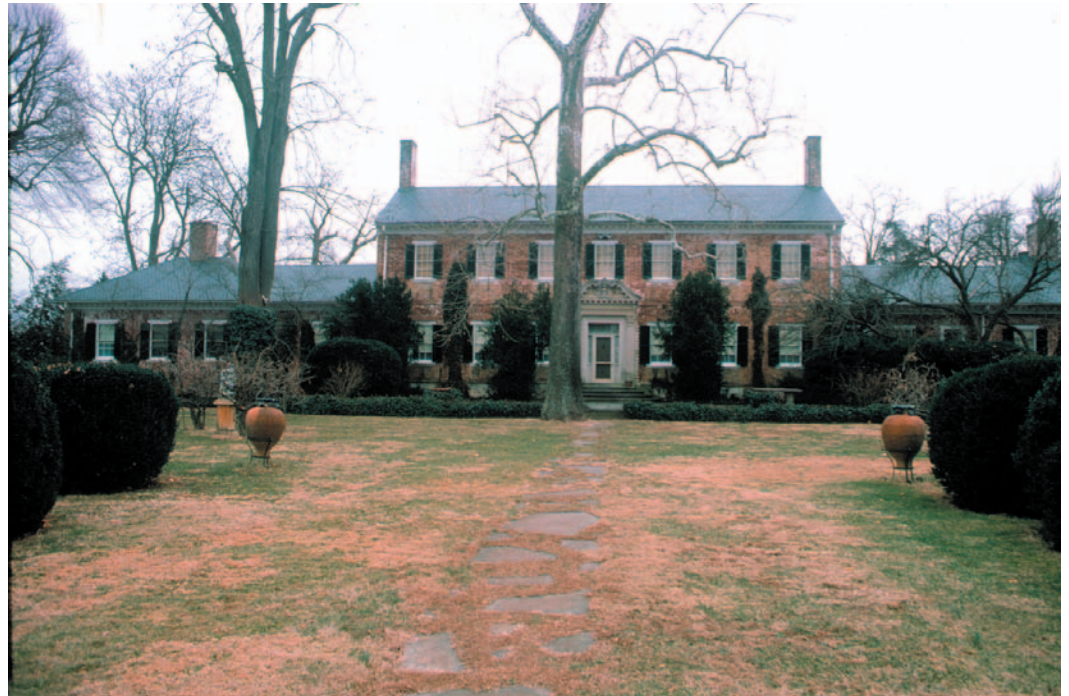
Fig. HH: East side of Chatham, circa 1975. (National Park Service)
