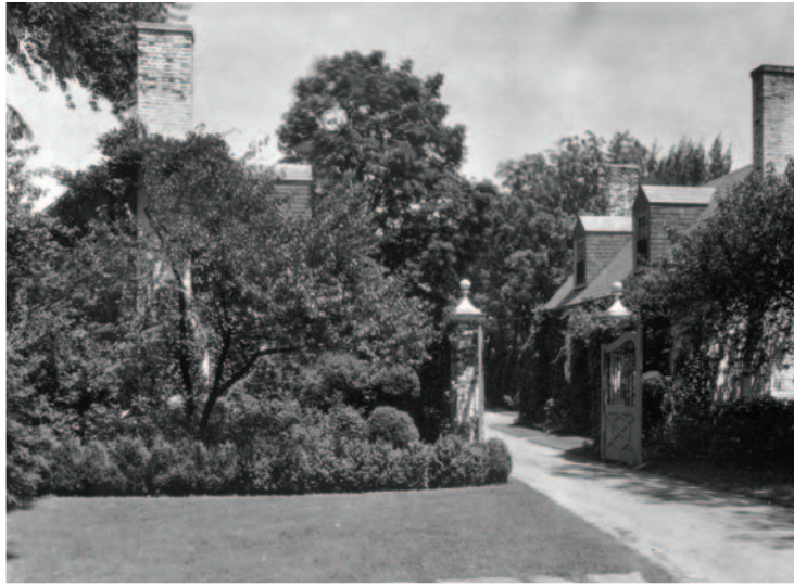
Fig. 51: Two outbuildings (kitchen on left and outbuilding #3 on right) from the west lawn looking northeast.
