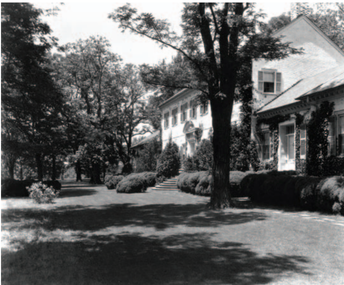
Fig. 6: Front of Chatham looking north with a locust tree (removed).
