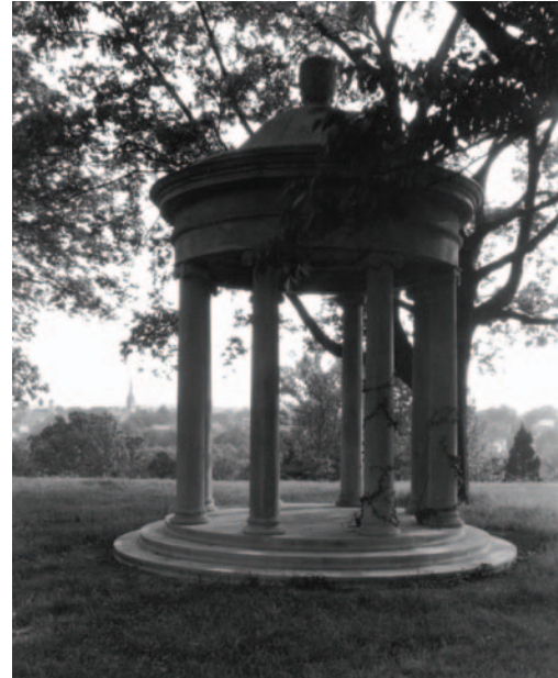
Fig. 9: Temple on lawn looking towards Fredericksburg without Pan.
