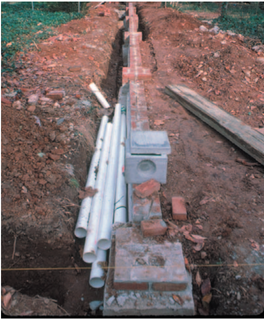
Fig. II: South garden wall restoration. (Reed Engle)
