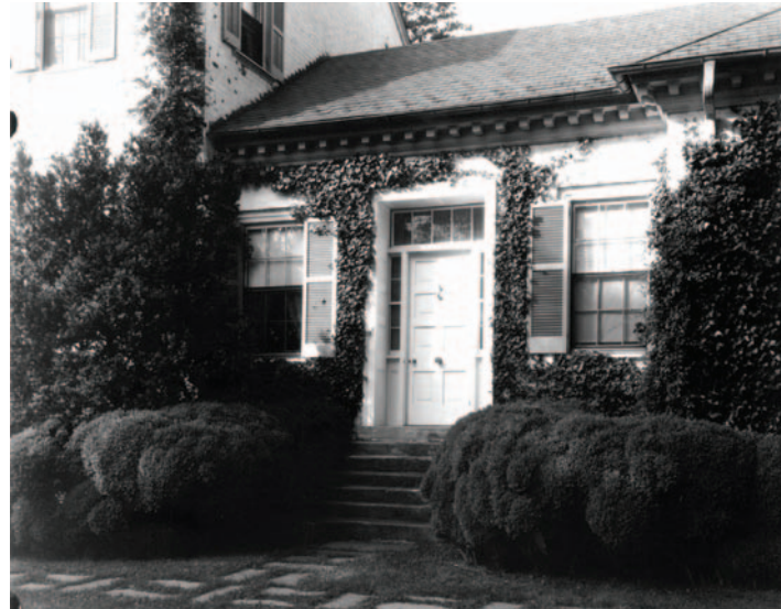
Fig. 5: Front of Chatham with door to southern hallway, looking northeast.
