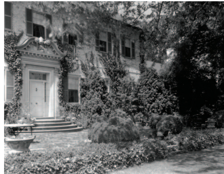
Fig. 13: Door and stone terrace along east side of Chatham, looking west.
