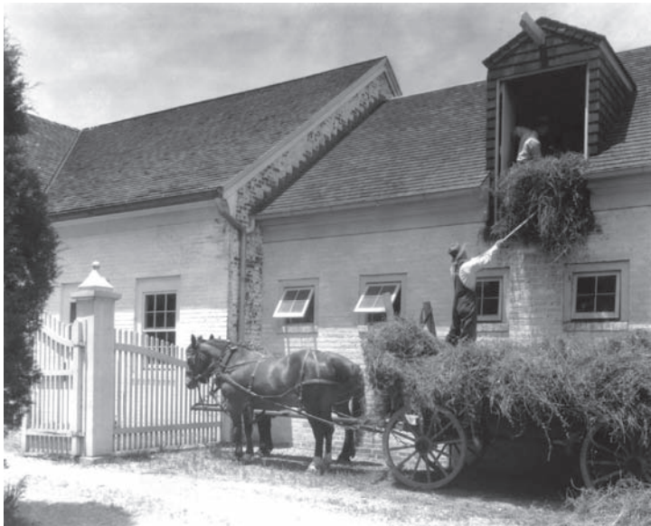
Fig. 61: View of hayloft and workers on far east side of garage looking west.
