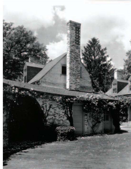
Fig. 54: Outbuilding #3 with chimney, dovecote, and kitchen on far right from service yard looking southwest.
