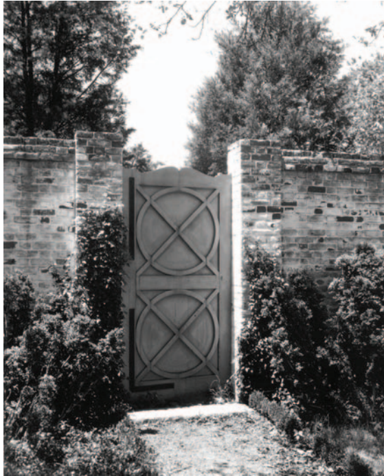
Fig. 45: On the east side of the east garden wall looking southwest towards a garden gate.
