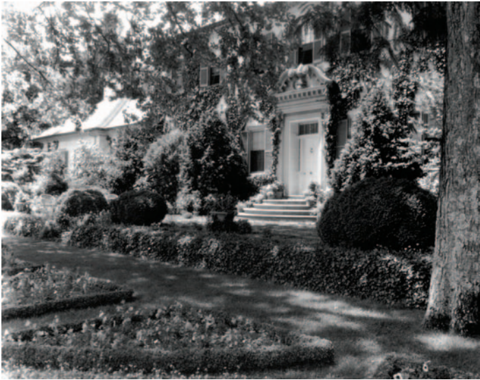
Fig. 14: Door and stone terrace with parterre in foreground and removed cedar looking south.
