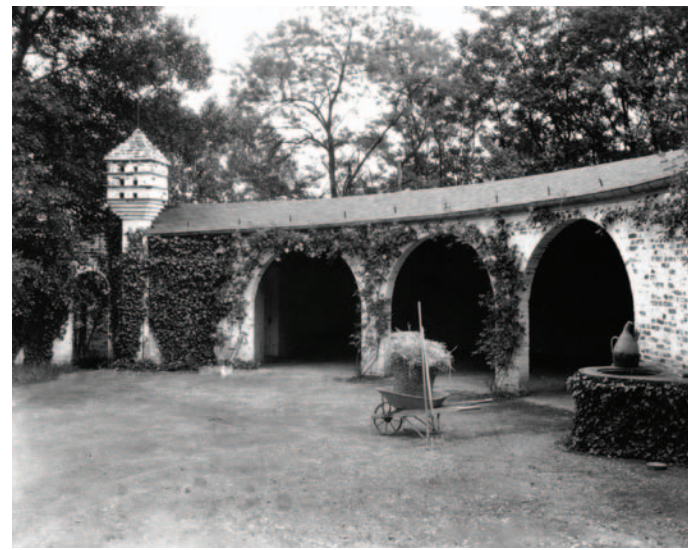
Fig. 56: Curved garage and Shipman-inspired dovecote in service yard looking southeast.
