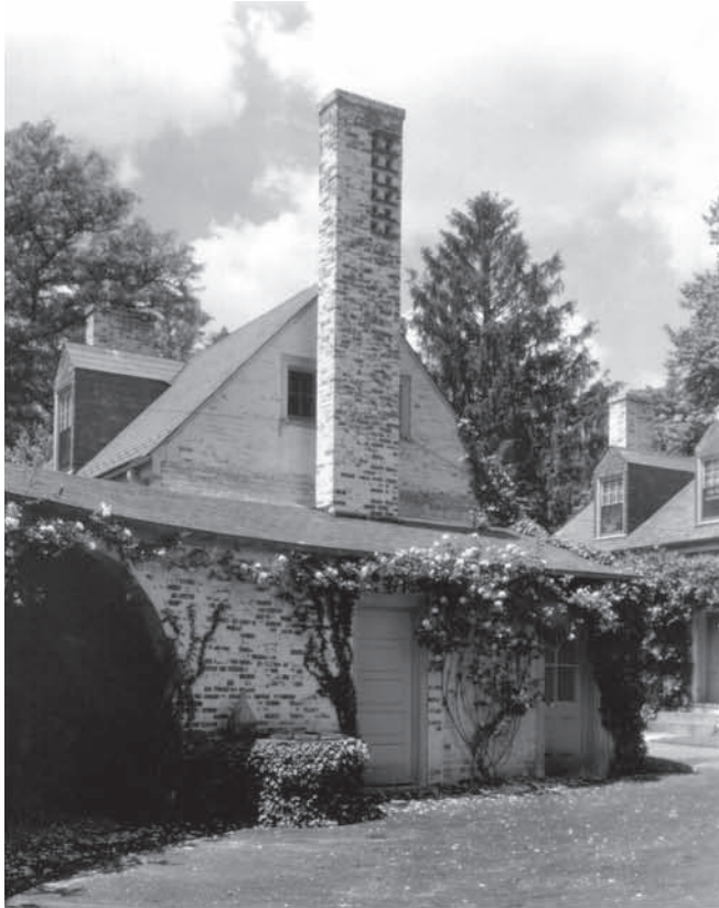
This view from the service yard of outbuilding #3 and the kitchen shows a Shipman-inspired chimney dovecote. John Pratt removed the dovecote and filled in the archway of the garage to accommodate a heating and cooling system for Chatham.
