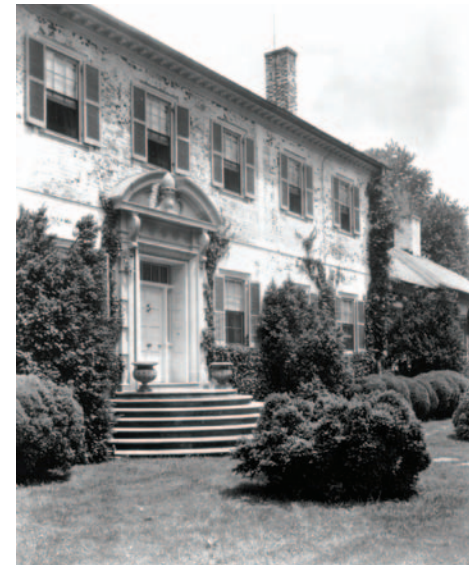
Fig. 1: Front door looking east with extensive boxwood planting.
