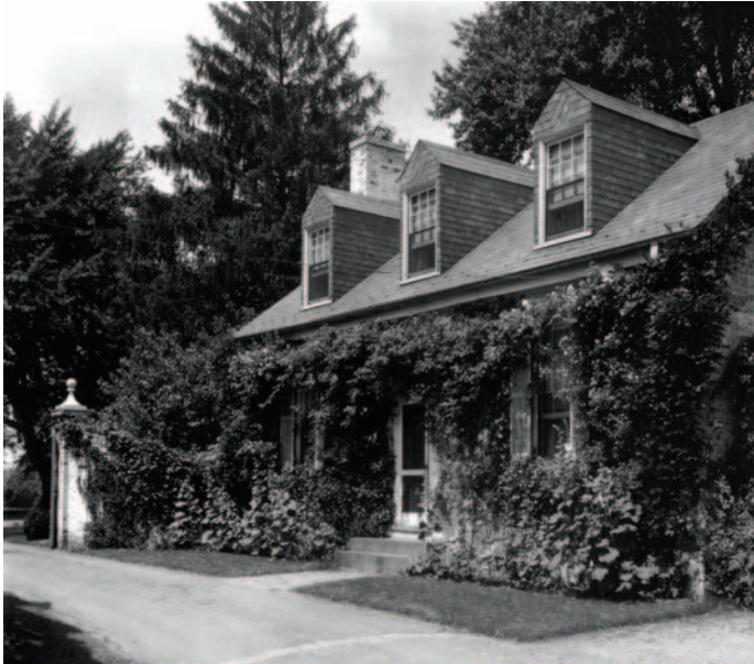
Fig. 53: The kitchen from the service area looking southwest.
