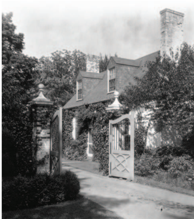
Fig. 52: Outbuilding #3 from west lawn looking east through wooden gate.
