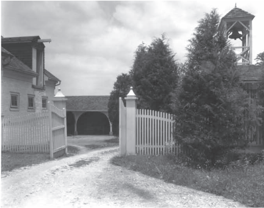
Plantings along the southern edge of the service yard have grown to form a dense woodland barrier on the edge of the property. In July of 2006, the wooden fence and gate were removed by the NPS to accommodate large delivery vehicles arriving at Chatham. The bell-topped corncrib is hidden western red cedar plantings.
